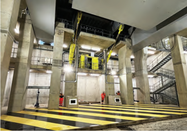
This perspective of the bridge shows the bascule pit and the rear underside of the bridge. The central hydraulic power unit actuates the two pairs of yellow cylinders efficiently
