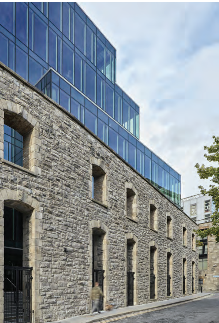
The Bow Street boundary wall incorporated into the completed development (facing north)
