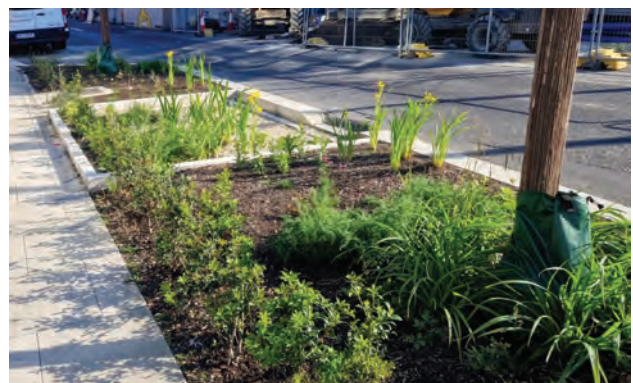
SuDS bioretention area
