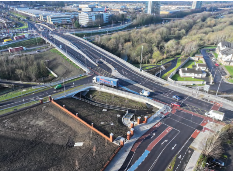
New pedestrian and cycle underpasses providing a fully segregated option for active travel users
