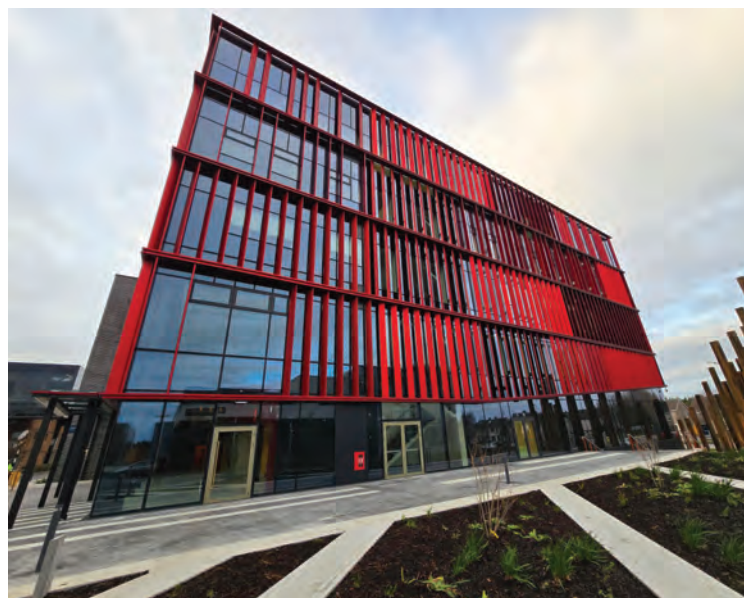
Side view of Polaris building façade
