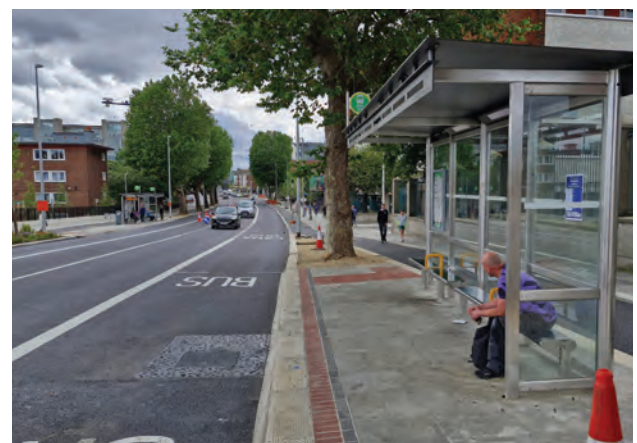
Extensive road and footpath reconstruction was required
