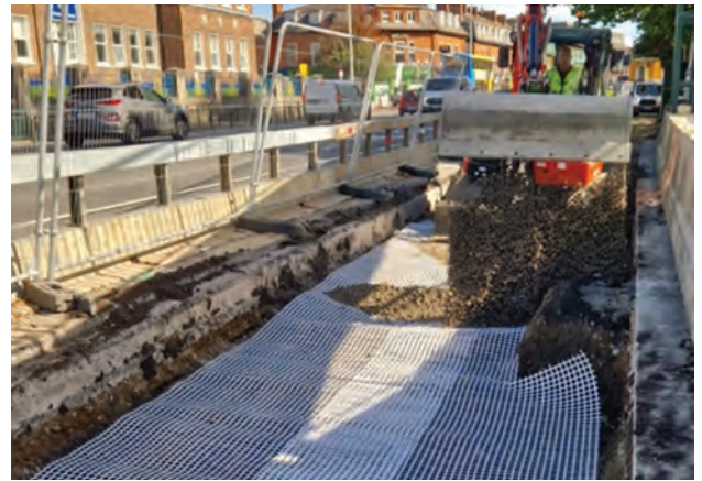
Image showing the upgrading and repaving of road and footpath pavements
