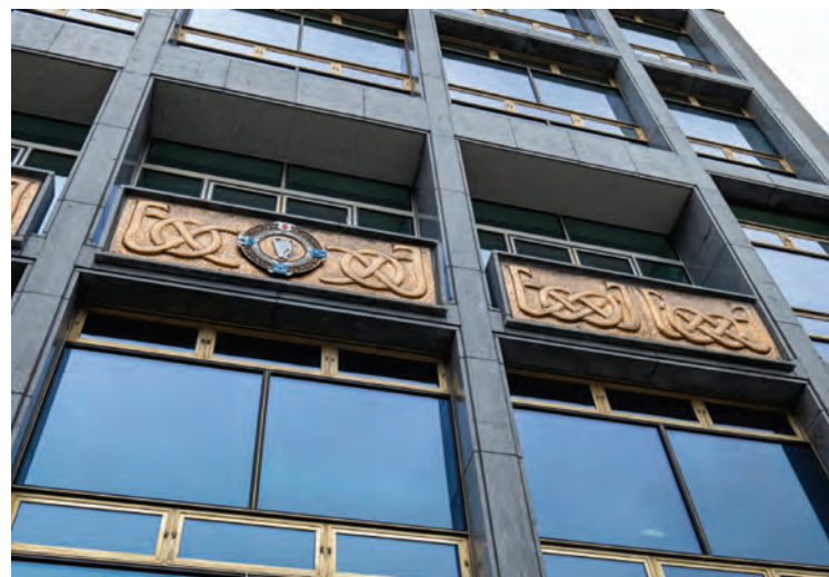
Refurbishment of protected façade
