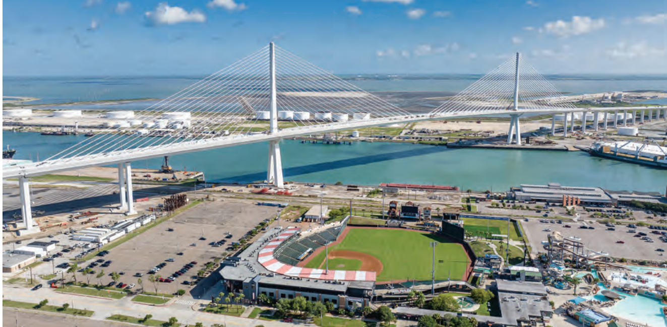
The completed bridge in June 2025. Image courtesy of Harbor Bridge Project
