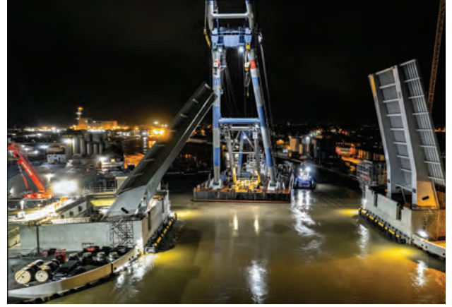
A drone photo of Herring Bridge during construction. The 1800-tonne, floating, sheerleg crane sits in the channel after placing both bascule leaves
