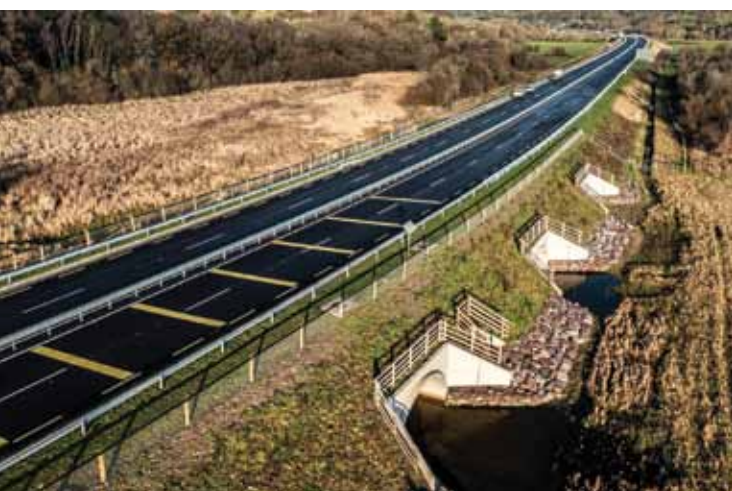
Flood culverts between River Sullane and Inniscarra Reservoir at the eastern tie-in of the scheme
