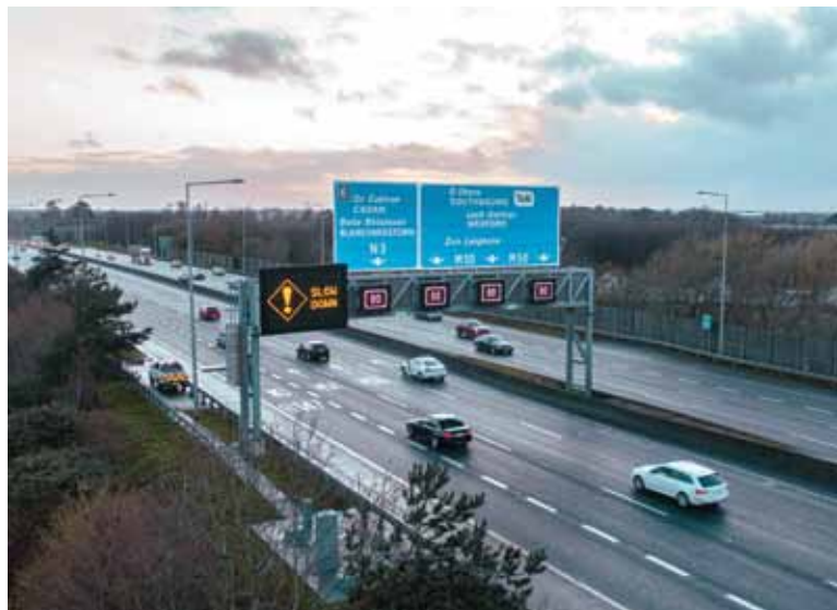
View of a gantry displaying speed limits and associated messaging to drivers
