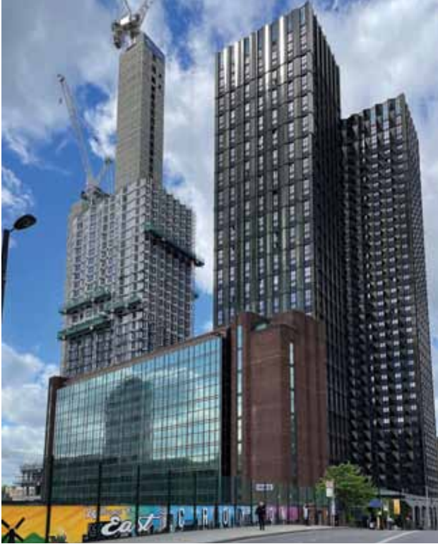
Module installation level 32
