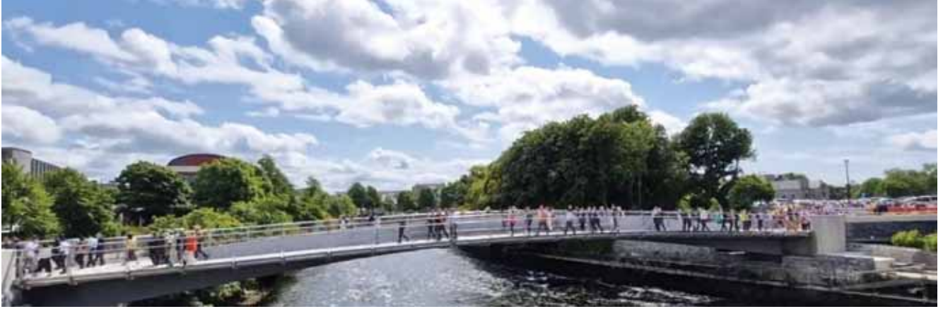
Spanning 51m, the bridge's semi-elliptical arch with a steel central spine beam and transparent handrailing creates an illusion of the bridge hovering over the river © Arup
