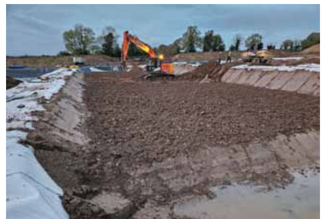
Placement of soil in Pond 2 with formation of the deep-water zone visible in the foreground
