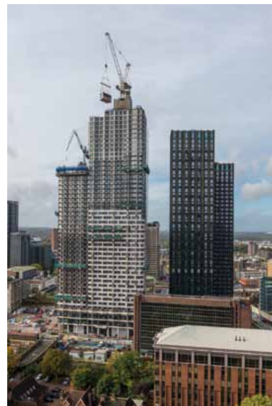
Module installation Level 48
