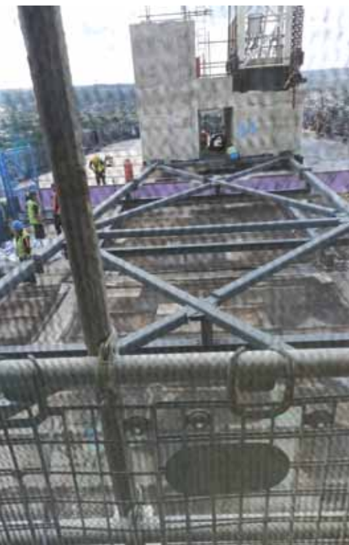
Level 35 temporary tie frame between cores
