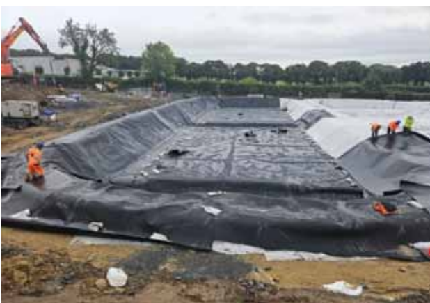
Liner installation in Pond 1, in foreground, with installation of protective geomembrane in Pond 2, shown in right background
