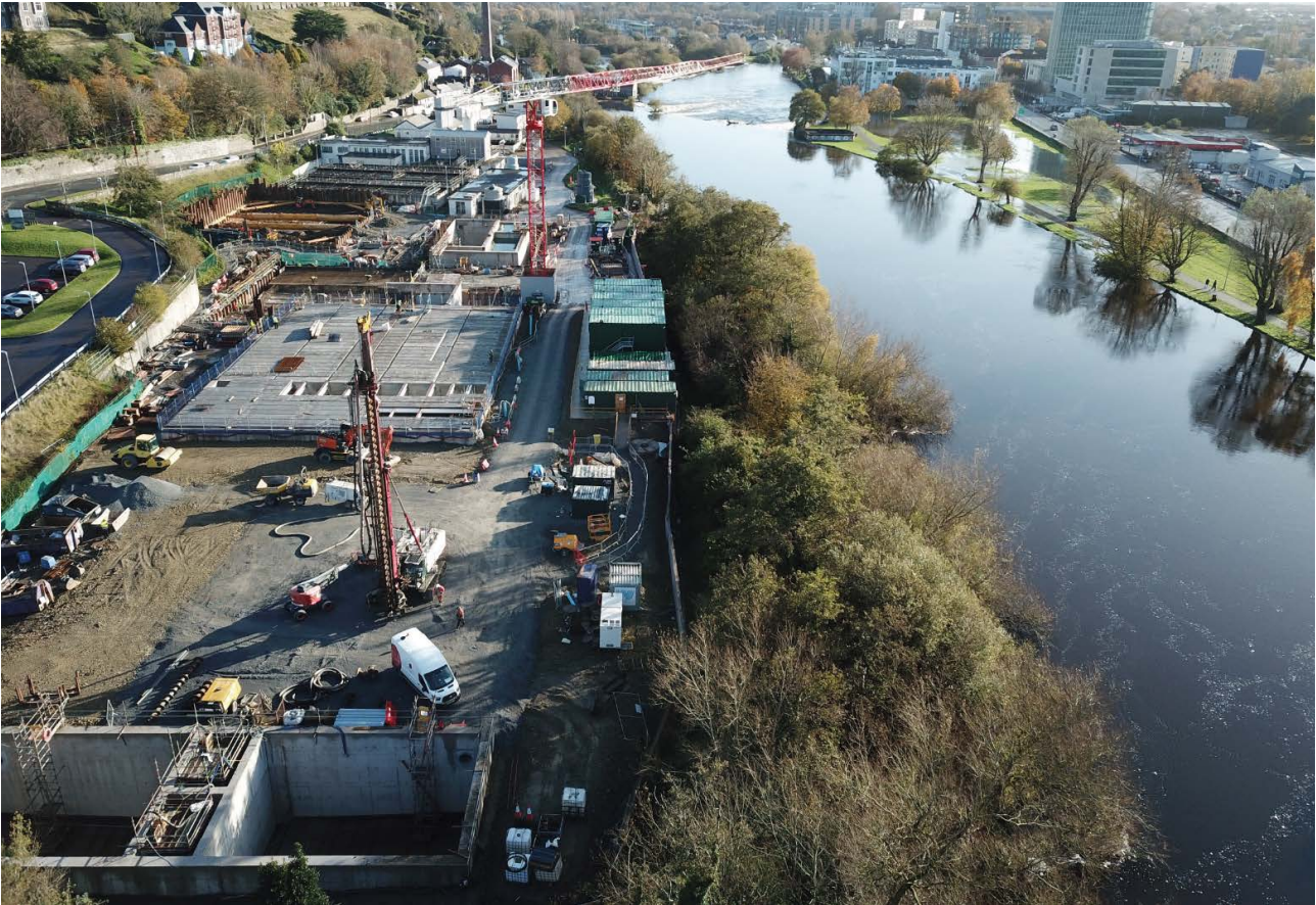
Lee Road Cork Courtesy of Irish Water/Uisce Éireann
