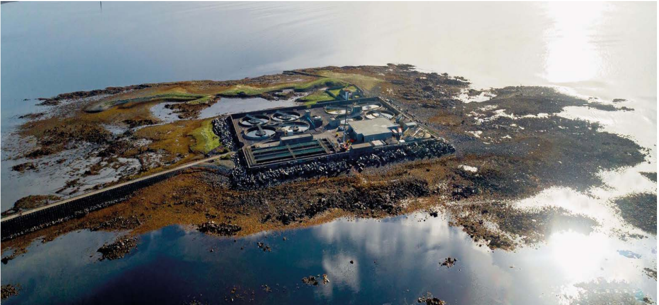
Mutton Island wastewater treatment plant, Galway Bay Courtesy of Irish Water/Uisce Éireann
