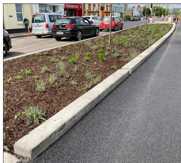
Figure 4.2: Median containing a rainwater garden designed to intercept rainwater on the way to a more conventional drain.
