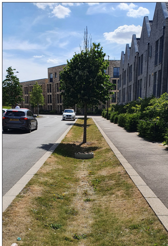
Figure 4.6: Swales should be designed with gentle slopes to facilitate ease of maintenance with positive drainage provided to prevent long-term ponding.
