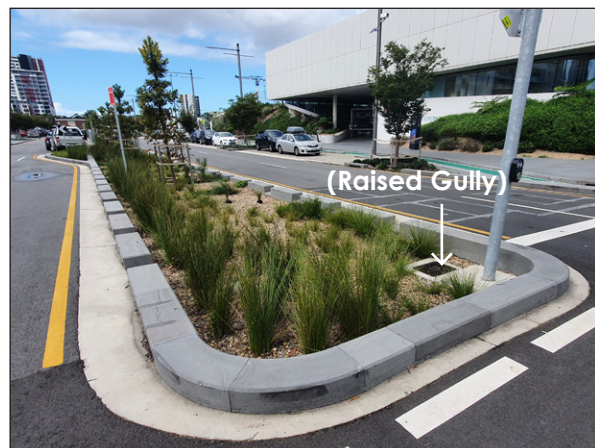
Figure 4.1: Verge (top) and median (bottom) designed as SUDs features. Note both features include an overflow drain into a more conventional system should the feature become saturated.
