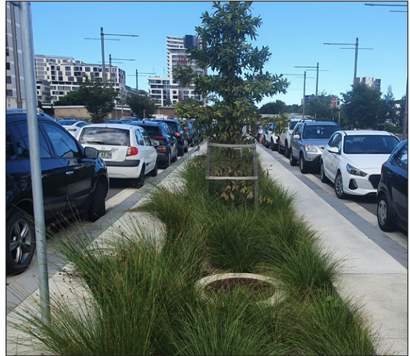
Figure 4.11: A wide edge is provided between parking and a swale to ensure clear access to vehicles.
