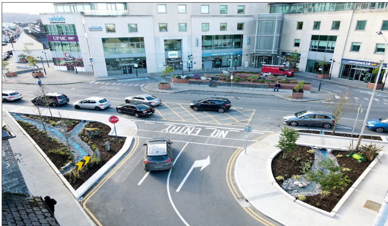
Figure 2.1: Bioretention Areas (Rain Gardens) – Pollerton Road/Green Lane Junction, Carlow. Carlow County Council
