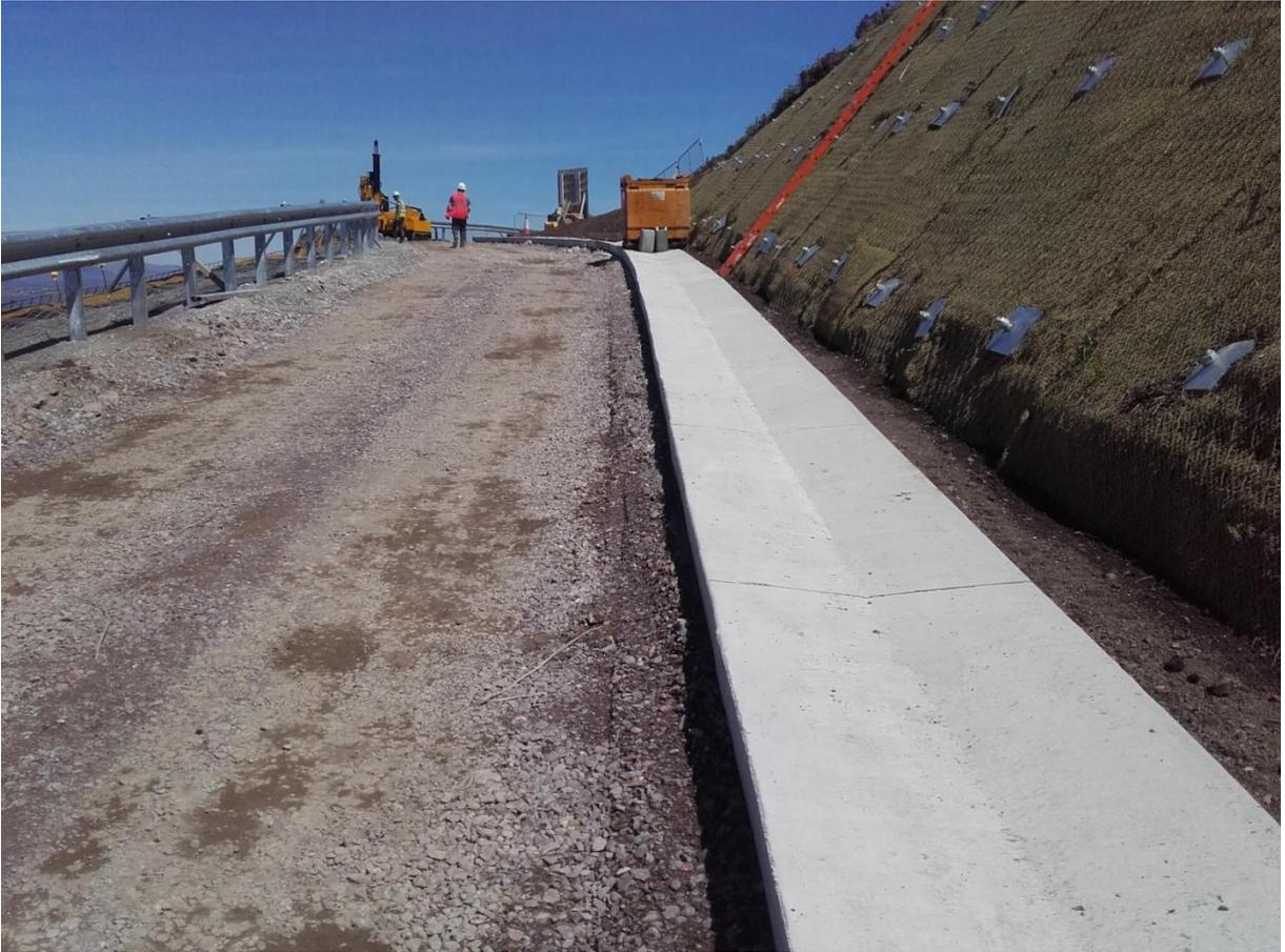
Figure 9 - Drainage channel
