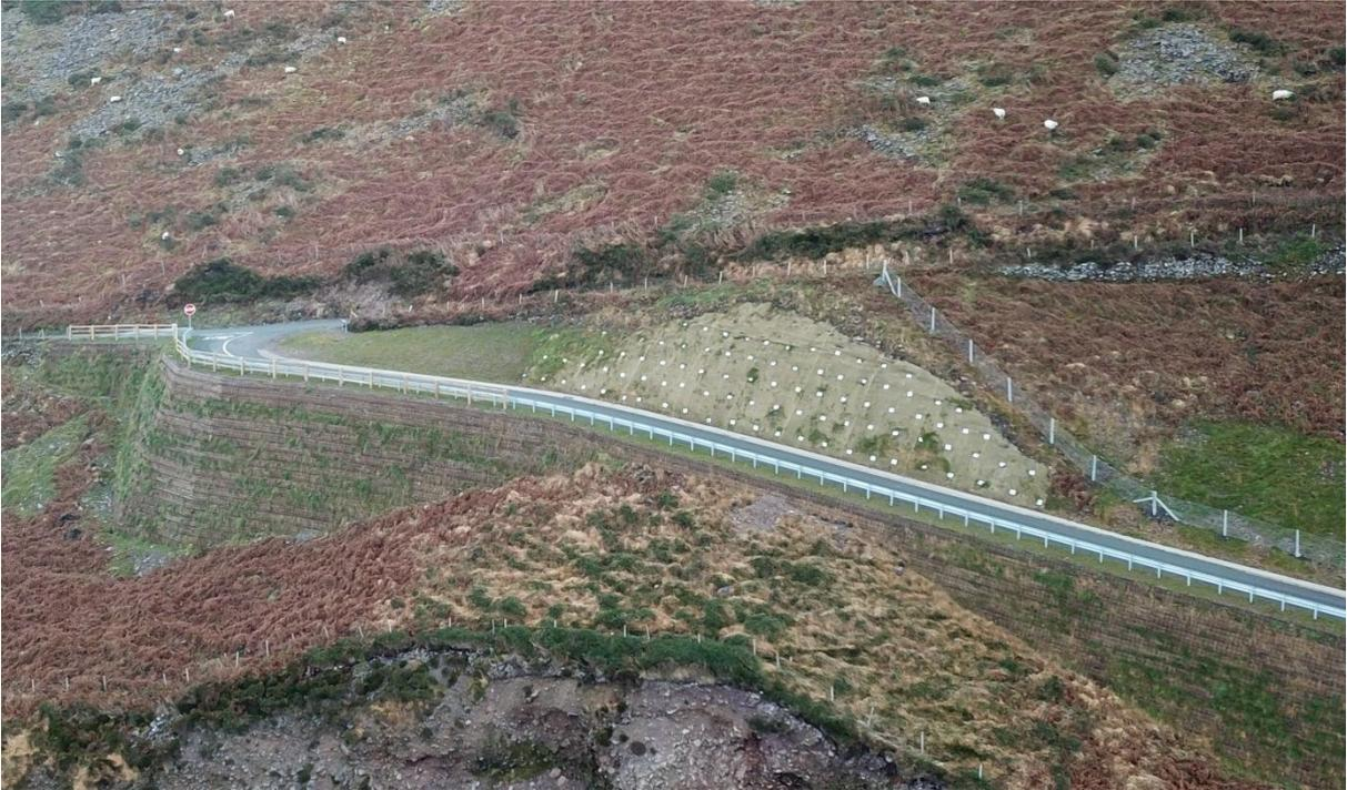
Figure 6 - Soil nailing at cut section below existing road
