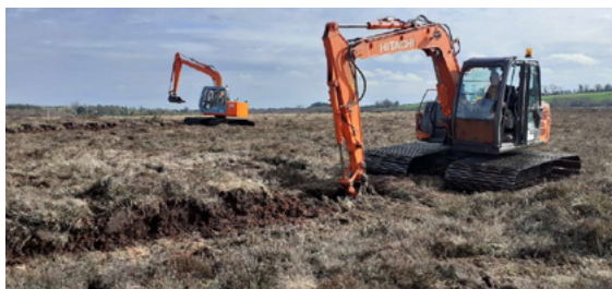
Contour bunding on Knockacoller bog Special Area of Conservation, Co. Laois
