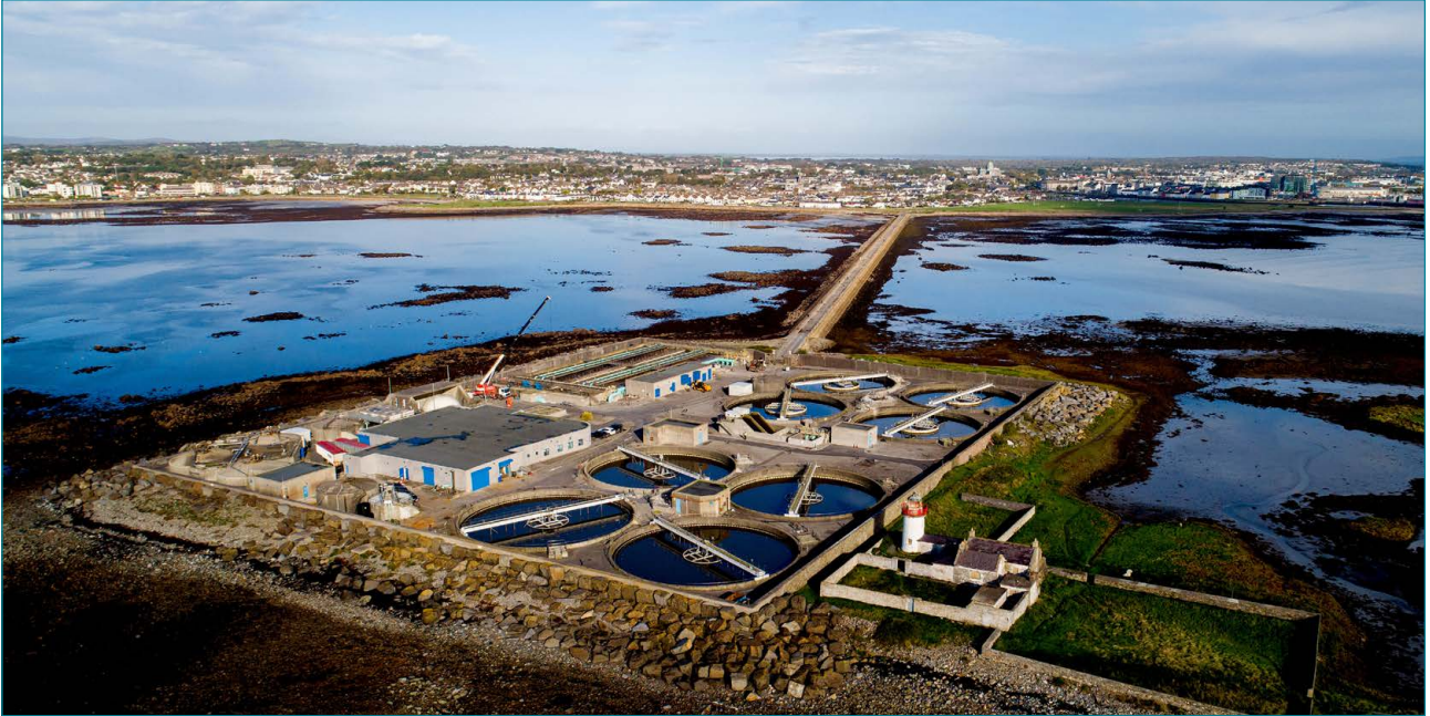
Mutton Island Wastewater treatment plant, image courtesy of Irish Water
